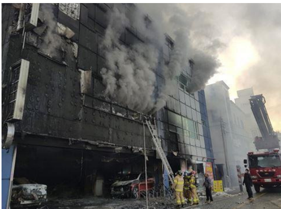
Fig. 1. Jecheon Sports Center Fire
