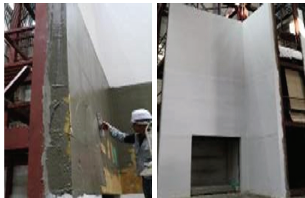
(c) Installation of Glass Fiber Mesh on Insulation (d) Finished EIFS
