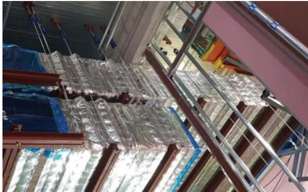
Fig. 2. Sprinkler Installation in Duct Site of the Picture
