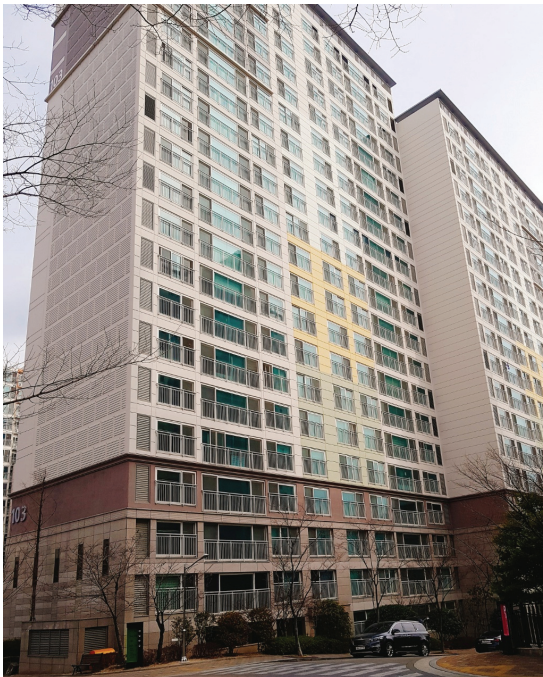
Fig. 1. The Exterior Wall of Apartment
